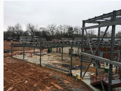
Steel Erection at Kitchen & Lobby
