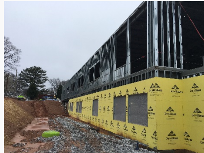
Exterior Sheathing & Framing
