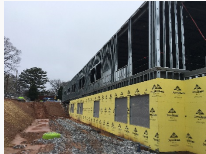
Exterior Sheathing & Framing
