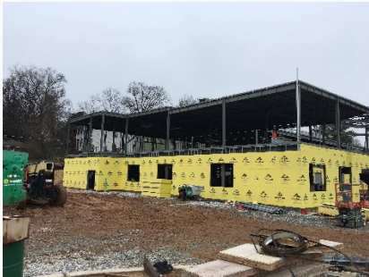
Exterior Sheathing & Framing
